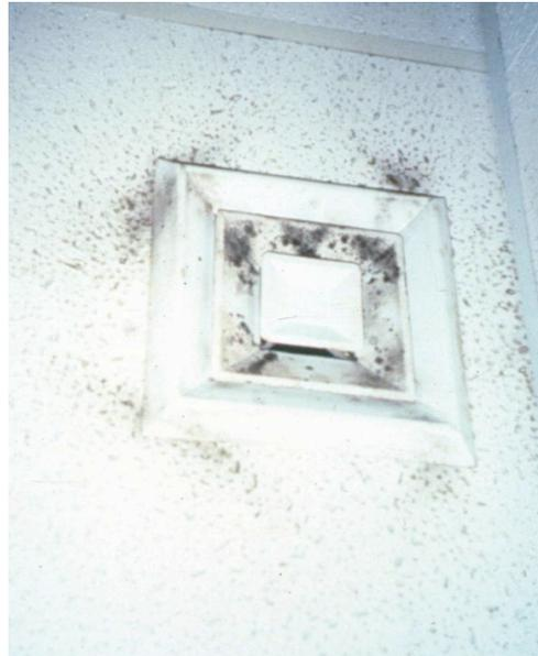
Second, the Coanda effect, which is the tendency for a fluid stream to stay attached to a convex surface, is exploited to increase the throw of air. The supply air discharged from the diffuser is caused to “stick” to the ceiling for some distance before detaching.
